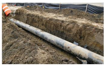
Support gas pipelines during excavation and backfill activities to avoid pipes being damaged by their own weight or soil compaction. Notify National Grid whenever cast-iron gas pipe is exposed or falls within an excavation trench's angle of repose.
