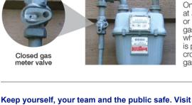
at a service meter or appliance. A gas valve is closed when the valve lug is perpendicular, or crosswise, to the gas pipe.
