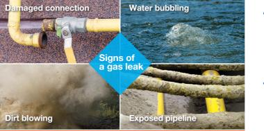
Leaking natural gas may throw dirt up into the air, kill grass or plants, or make bubbles in water. A damaged connection to a gas appliance and/or pipelines exposed by fires or floods may be sources of leaks.
