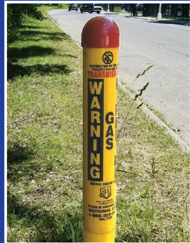
Natural gas pipeline markers are generally yellow and black. They're placed near pipelines but not necessarily directly on top of them.
