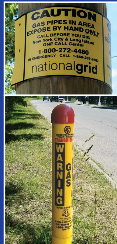
Natural gas pipeline markers are generally yellow and black. They're placed near pipelines but not necessarily directly on top of them.
