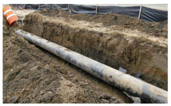
Support gas pipelines during excavation and backfill activities to avoid pipes being damaged by their own weight or soil compaction. Notify National Grid whenever cast-iron gas pipe is exposed or falls within an excavation trench's angle of repose.
