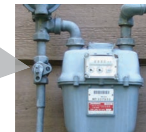
Closed gas meter valve
