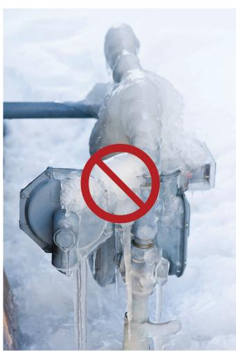
Heavy winter storms can compromise natural gas infrastructure, both aboveground and underground. Consider the possible impact of major snow and ice events on natural gas infrastructure when sizing up incidents involving natural gas leaks, fires or explosions.
