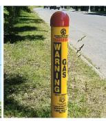
These markers are meant only as a general guide and warning and do not mark a pipeline's precise location or depth. You can also locate pipelines in your area by warning the process of t You can also locate pipelines in your area by visiting the National Pipeline Mapping System website at https://pvnpms.phmsa.dot.gov/PublicViewer.
