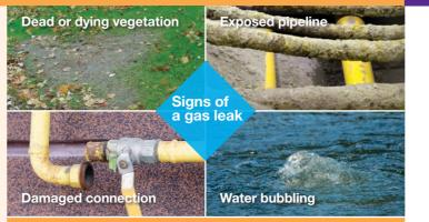
Leaking natural gas may kill grass or plants, throw dirt up into the air or make bubbles in water. Pipelines exposed by fires or floods may be sources of leaks, as may a damaged connection to a gas appliance.
