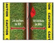
The tolerance zone varies from state to state. It is 24" in New York and 18" in Massachusetts. For your safety, use ONLY hand tools or vacuum technology within this zone. Always contact your state 811 center before digging and for the most current requirements.
