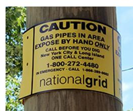
Pipeline markers are usually found where a high-pressure pipeline intersects a highway, street or railway and at other readily visible points along a pipeline right of way (ROW). A ROW is a corridor of land clear of trees, buildings or other structures—for example, alongside a railroad track.
