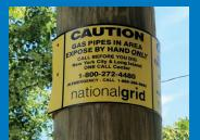
Many pipelines are underground in public areas. Line markers are sometimes used to indicate their approximate location but not depth. The markers display the name of the pipeline operator and the telephone number where the operator can be reached in the event of an emergency. These markers are usually freestanding; in urban areas, they may also be found on utility poles.
