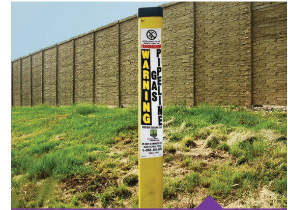
Natural gas pipeline markers are generally yellow and black. They're placed near pipelines but not necessarily directly on top of them.
