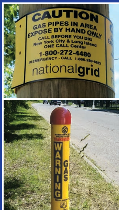
Natural gas pipeline markers are generally yellow and black. They're placed near pipelines but not necessarily directly on top of them.
