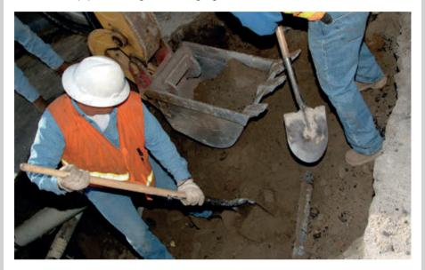
Buried power lines and natural gas pipelines can be easily damaged and are dangerous to contact. Before you can safely work close to an underground utility line with mechanized digging equipment, you must see the line with your own eyes:
