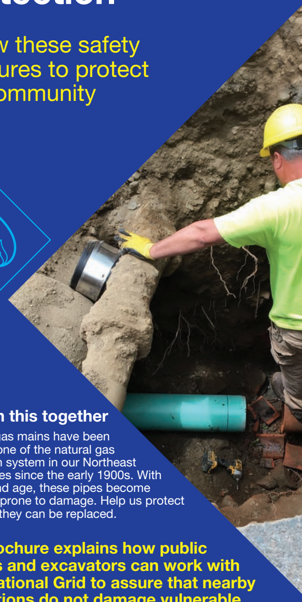
Cast iron gas mains are brittle and can break, endangering life and property when natural gas leaks.
